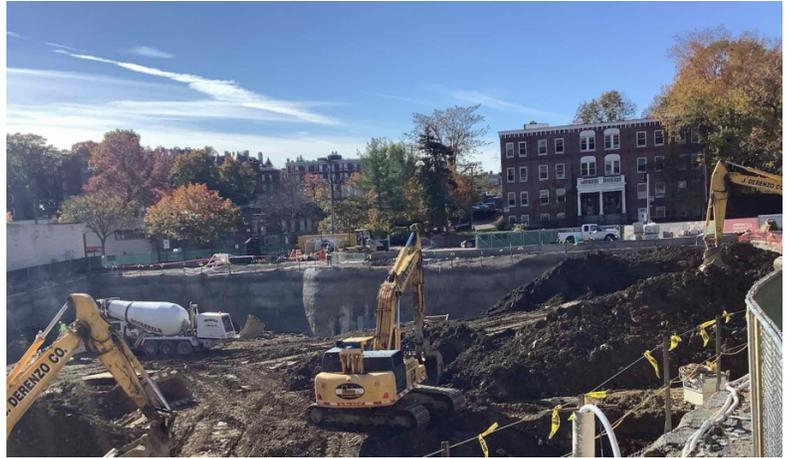
Soils hauling are approximately 75% complete, the final 20 – 25' cut down and hauling operations will continue after SOE is complete. (Photo Below)
